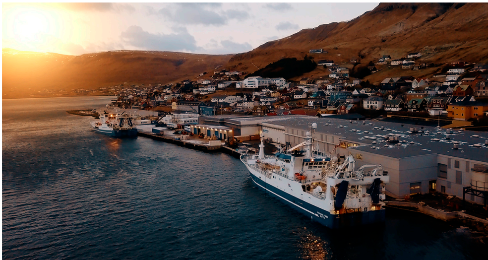
Fish processing factory Varðin Pelagic in Tvøroyri
